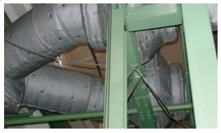
**DUAL 24" EXHAUST PIPING & CATALYTIC CONVERTER'S**
