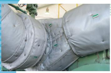
**ENGINE EXHAUST TURBOCHARGER**
