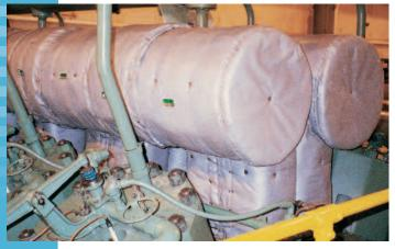
TCV-12 SECTIONAL MANIFOLD EXHAUST
