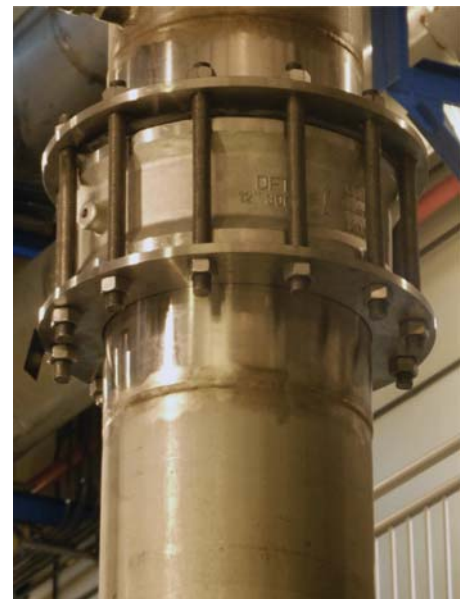
A close-up view of one of the 20 axial flow check valves installed at the membrane plant.
