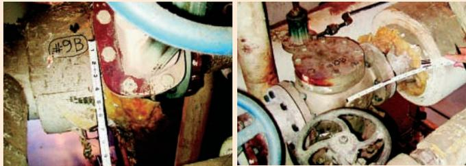
Valves & Fittings are Marked or Tagged & Measured for Design
