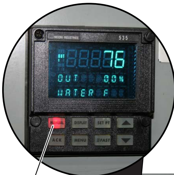
Heater in "AUTO" mode not running
