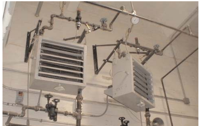
Armstrong Unit Heater Installation
