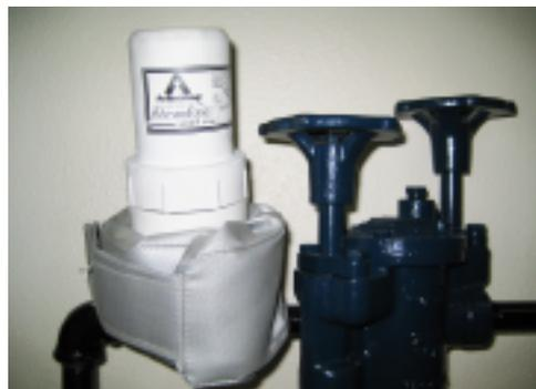
Figure 6. Insulation wrap installation
